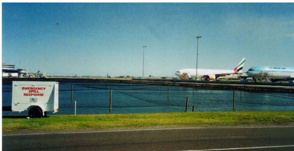
Bird netting over ponds at Sydney Airport
